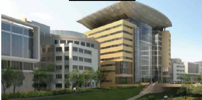
Main Central Site 7,000kW x 5
