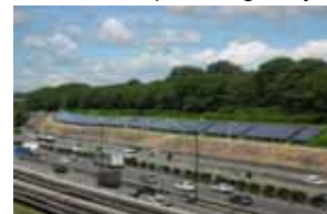
Roads: Slope in Highway
