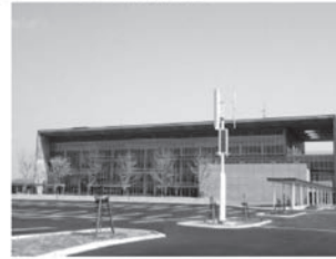
City hall in NIIGATA
