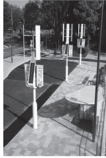
Station in OSAKA
