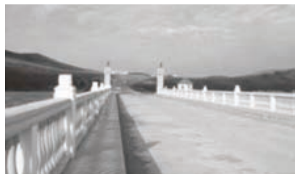
Photograph 4.1 Nomrog river bridge (Sumer BCP) with 340 meter length
