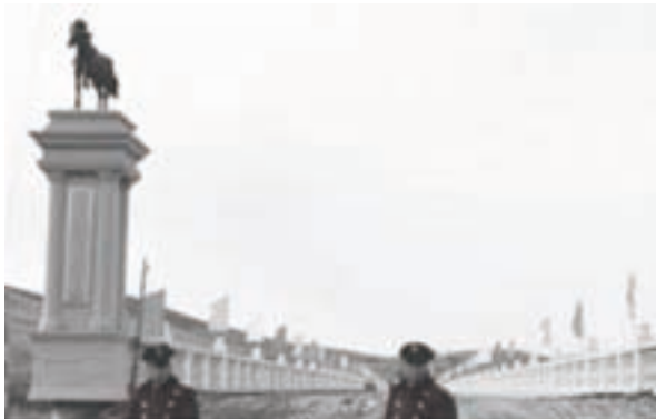
Photograph 3.7 The Bridge between Arxan and Sumber
