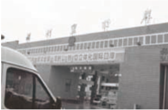
Photograph 3.6 Manzhouli Road BCP
