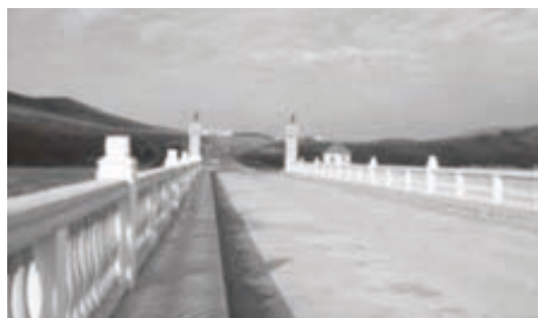
Photograph 4.1 Nomrog river bridge (Sumer BCP) with 340 meter length
