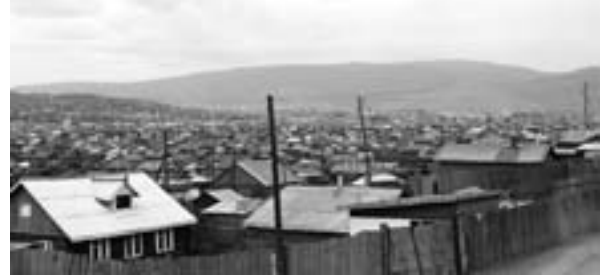
Photograph 1: Ger District in Ulaanbaatar City
