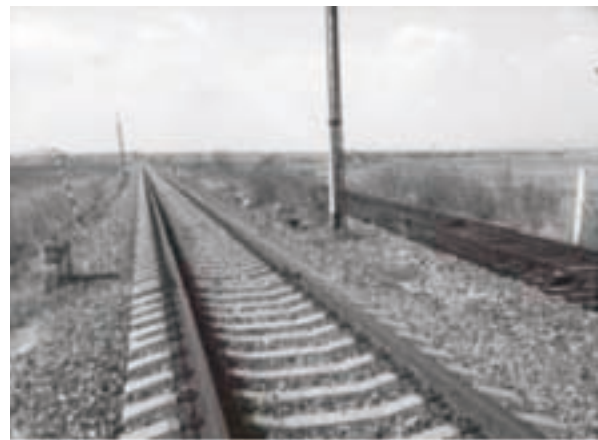
Photograph 1 Baranovsky - Khasan (left line to DPRK - to Khasan), right line - to China (to Kamyshovaya, out of operation)
