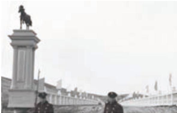
Photograph 3.7 The Bridge between Arxan and Sumber
